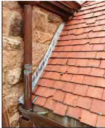
EXISTING COPPER FLASHING, GUTTERS, & DOWNSPOUT CONDITIONS
