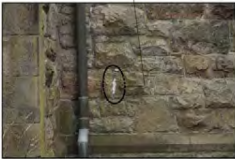
REMOVE THE CAULKING THAT WAS APPLIED TO MASONRY JOINTS TYPICAL
