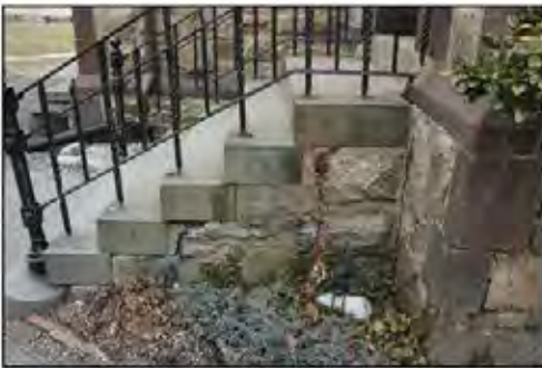
REPAIR STEPS AND THE GAP BETWEEN THE TOP LANDING AND THE CHURCH. NOTE THAT ALL THE TREADS HAVE MOVED OUT OF THE ORIGINAL POSITION AND WILL HAVE TO BE RESET.
