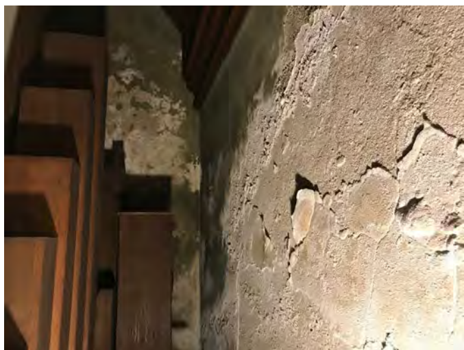
Wooden bass pipes; scaling, water-damaged chamber walls
