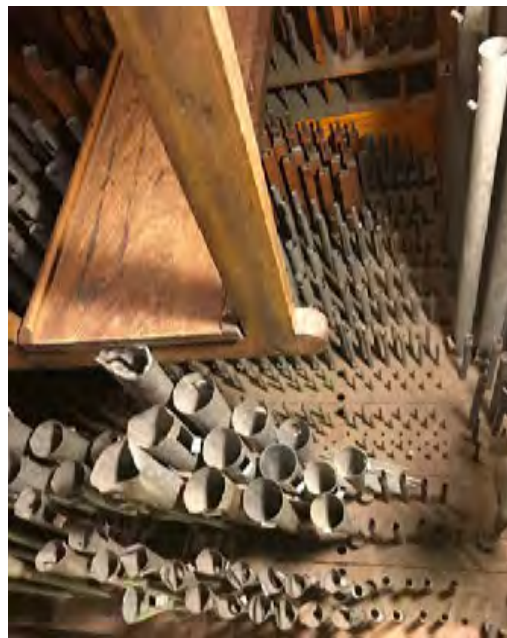
Damaged metal pipes in foreground
