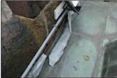
BELFRY ROOF: INSTALL NEW COPPER FLASHING AT ROOF TO WALL TRANSITIONS
